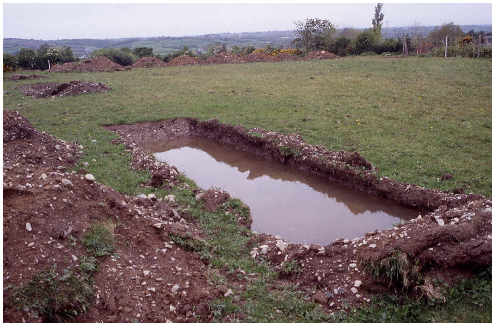
Plate Four: Trench B showing poor drainage of site (looking northwest)
