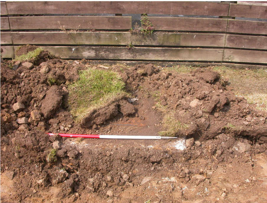
Plate 4: View of manhole uncovered along western edge of Trench A.
