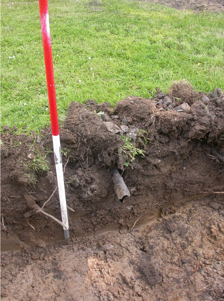
Plate 7: View of drain pipe at southern end of Trench A.
