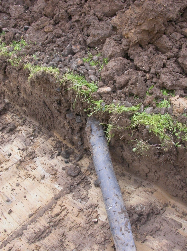
Plate 10: View of north-west to south-east aligned drain in Trench B.
