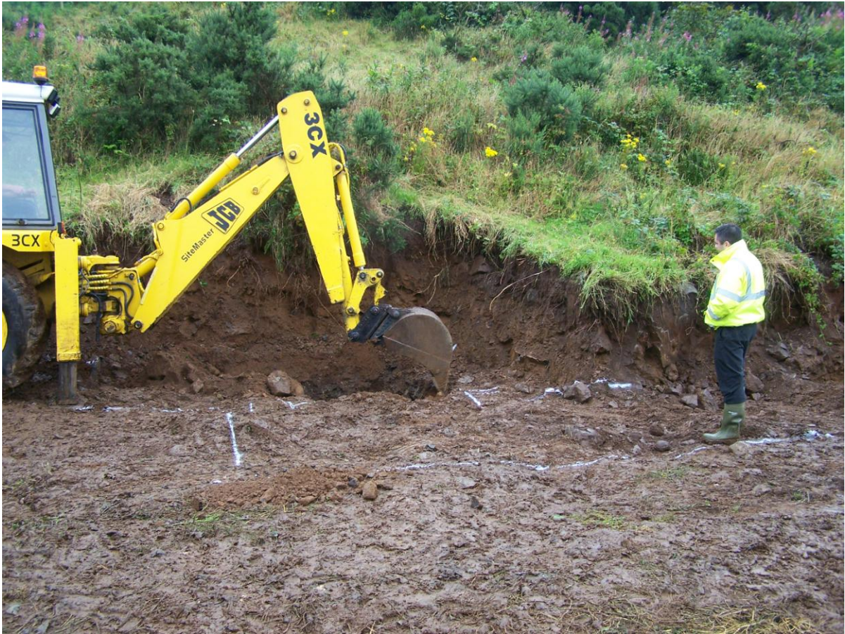
Plate 4: Excavation of the service trench, looking north.
