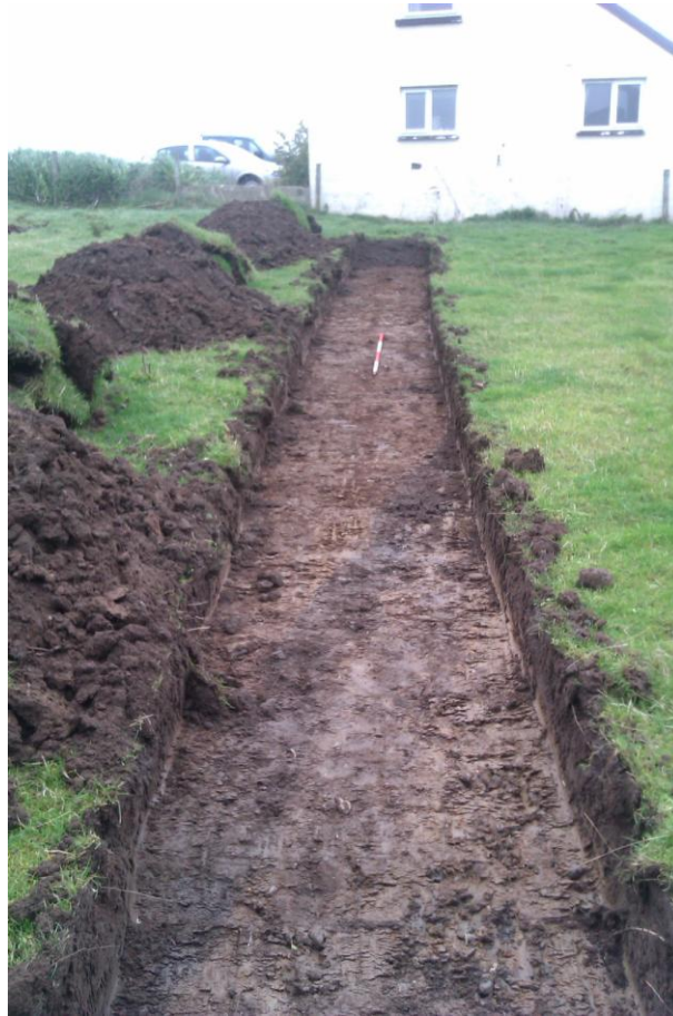
Plate 13: Trench 5 following removal of upper deposits, looking west
