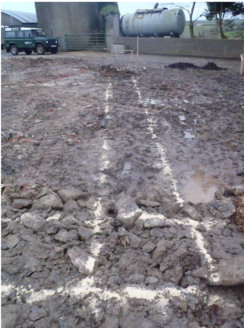
Plate 29 Northeast facing view of site pre-excitation of foundations
