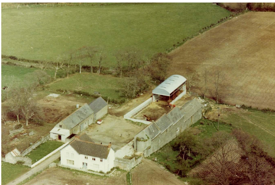
Plate 2 Aerial view of Inishargy House, yard and out-buildings, looking northeast, dated 1966. Church ruins visible on the left (photo: landowner's personal collection)
