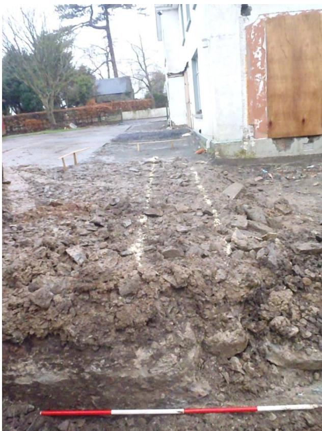
Plate 34 Northwest facing view along line of house and fifth foundation cut
