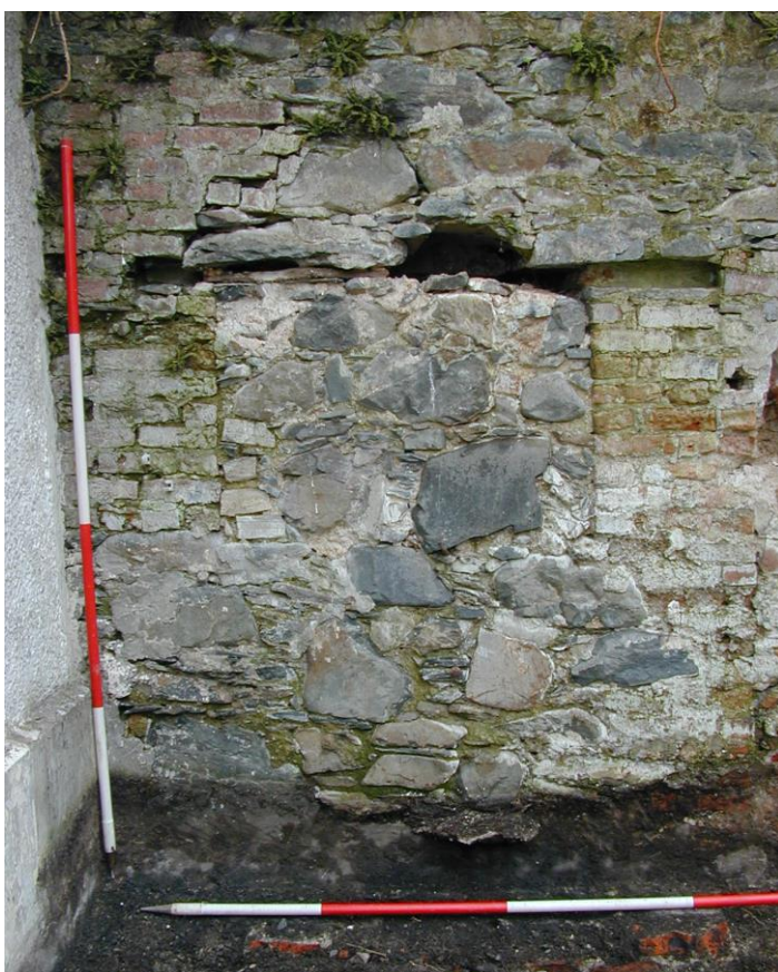
Plate 10 Northeast facing view of blocked up oven in 17 th century cross wall
