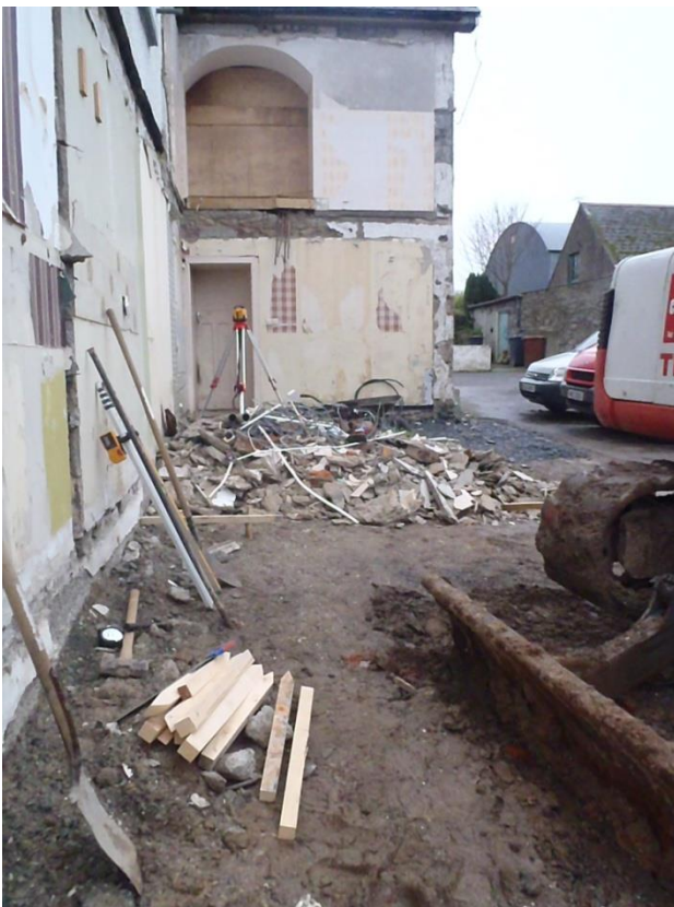
Plate 16 Northwest facing view of Inishargy House post removal of extensions
