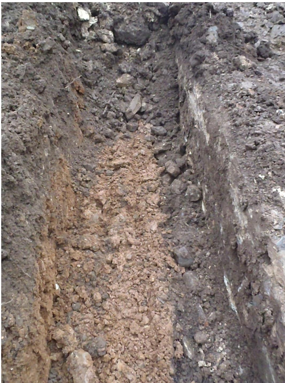
Plate 30 Southwest facing view of fourth foundation cut and uncovered wall, mid-excavation
