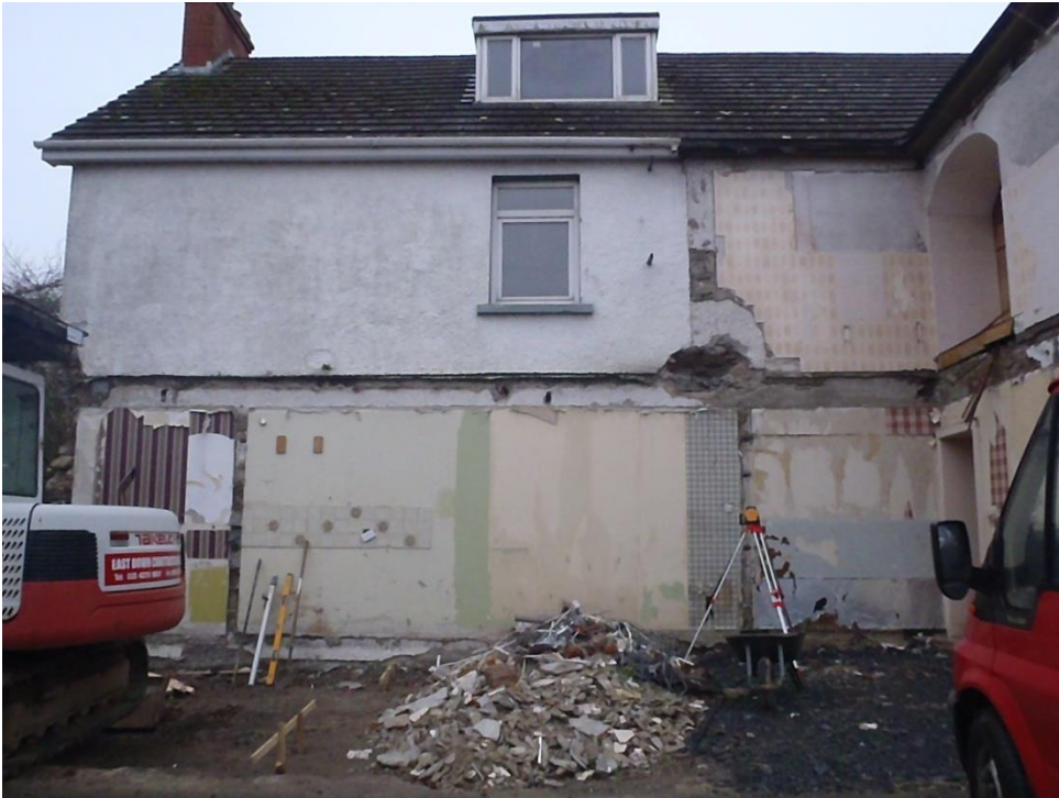
Plate 15 Southwest facing view of Inishargy House post removal of extensions
