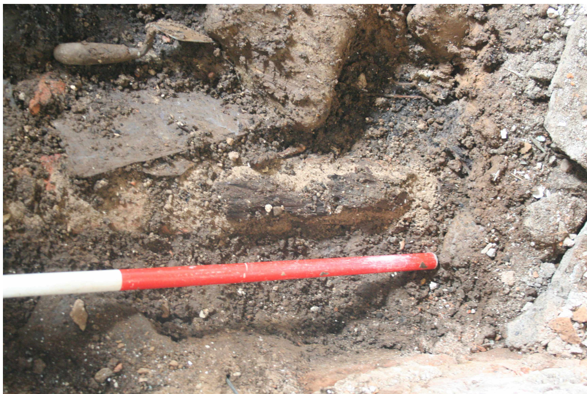
Photo 21: Remnants of wooden floor adhering to mortar on a brick joist support (413) in the extreme west of Trench 4.
