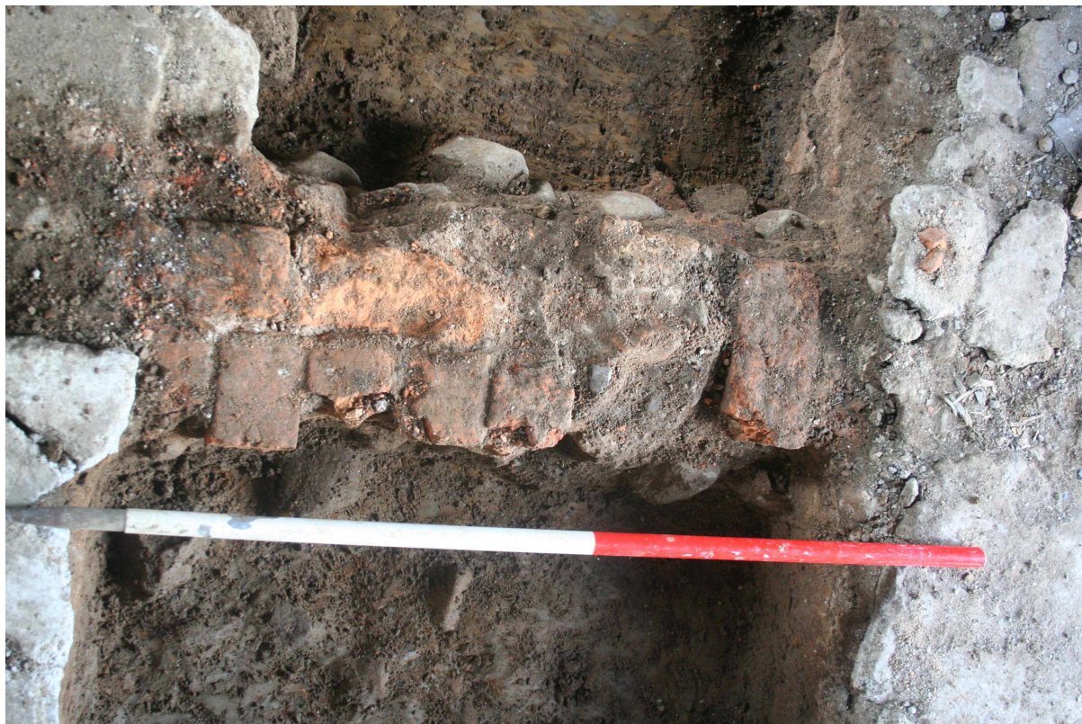
Photo 18: Photo of internal wall 404, brick courses still intact
