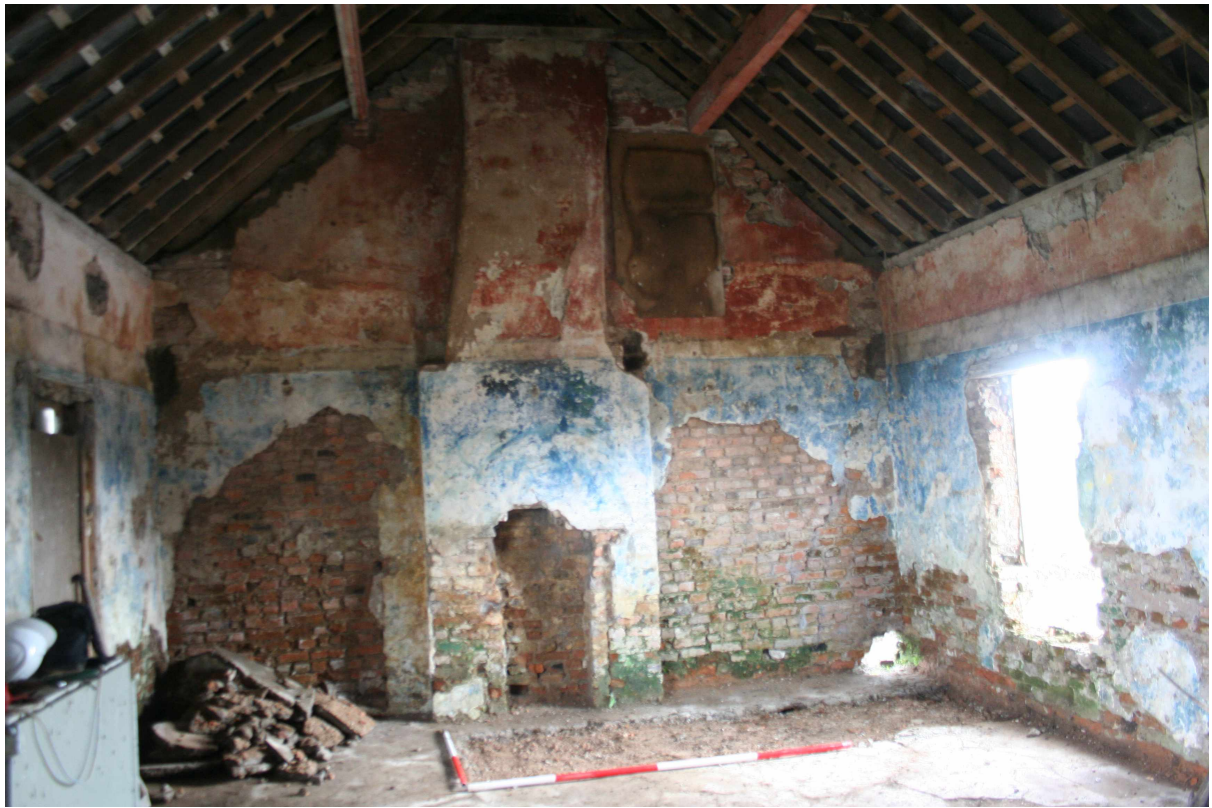
Photo 6: East gable and Trench 3 immediately after removal of concrete floor.
