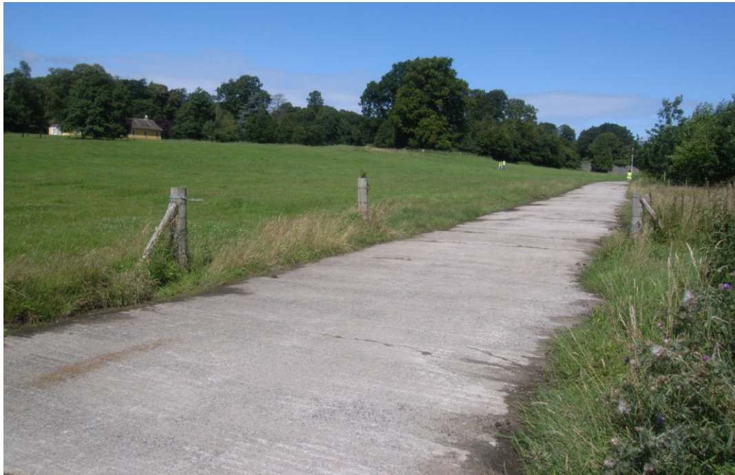
Fig. 6. Stretch of concrete road. Derrymore House at left (RIMG0005(2)).
