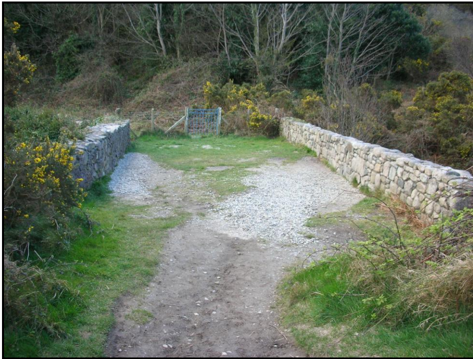
Figure 19: The medieval bridge over the Bloody Bridge River
