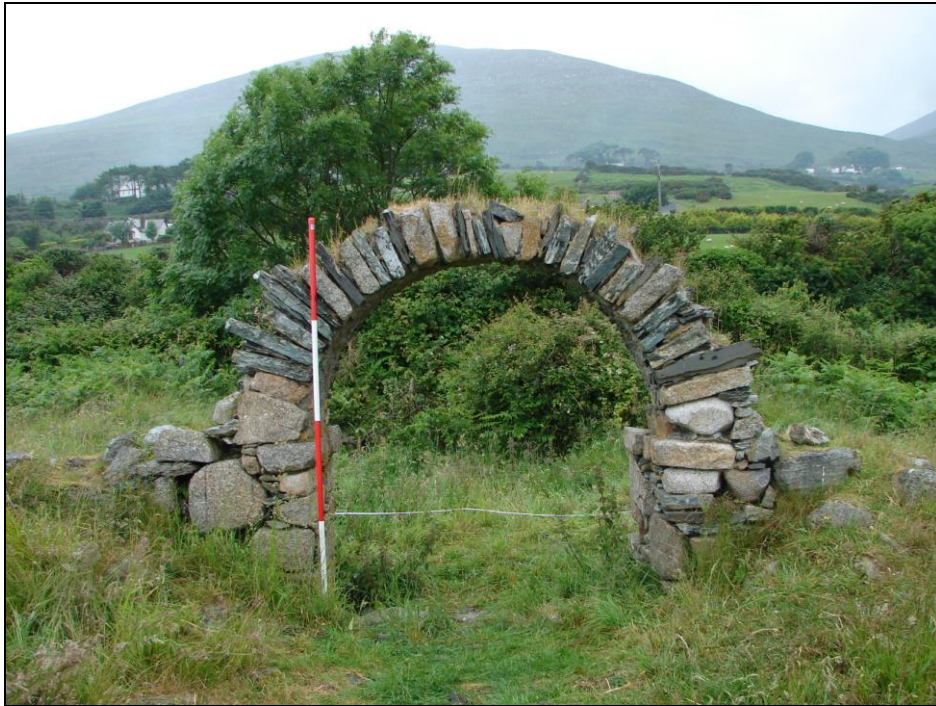
Figure 15: Chancel arch, looking west
