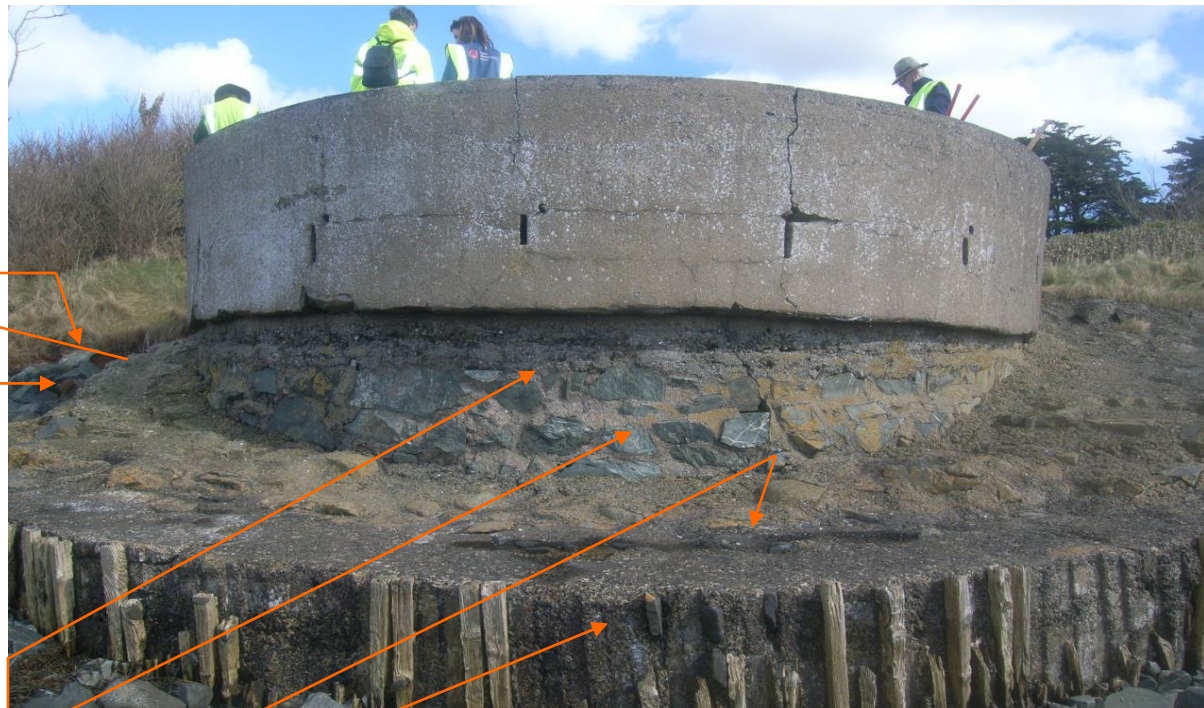
Fig 18 the summer house base foundation
