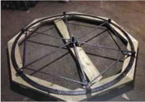
Figure 09: The chassis of a modern revolving summer house on which the wooden structure would be built. The original Mount Stewart one would have been very similar.
