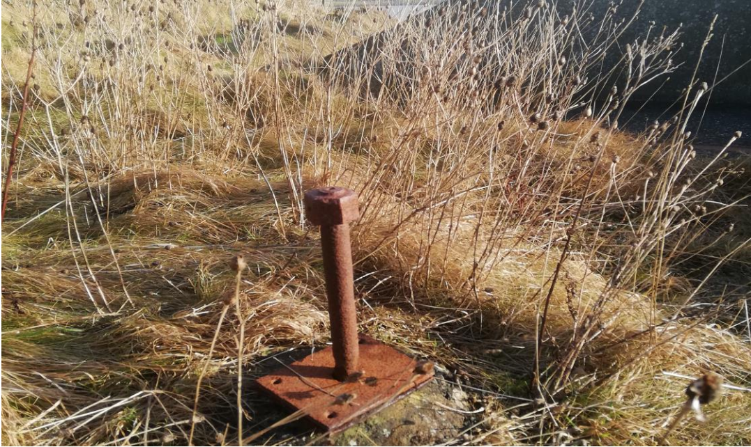
Fig 11 Close up of the central iron axle with a mounting plate
