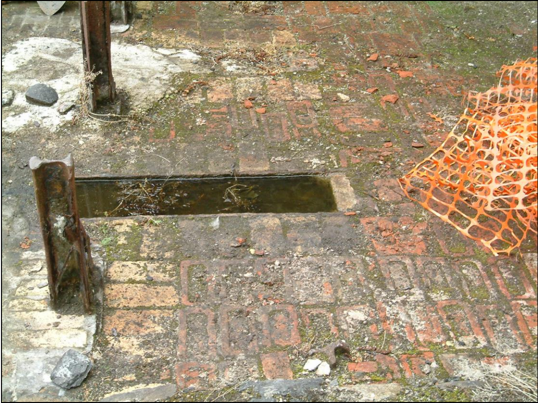
Fig. 42: Retort House floor from N showing northern pan and rails
